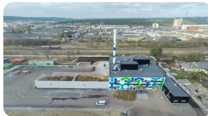
Biomass boiler house Vilnius (25 MW)
